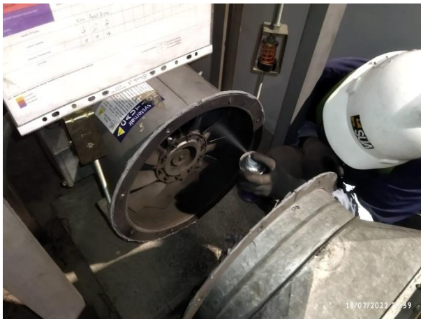
Perawatan unit Ventilation System
