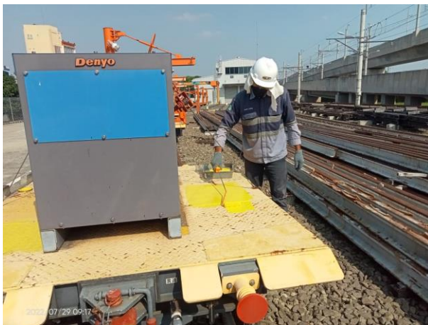
Pengecatan equipment Steel Trolley
